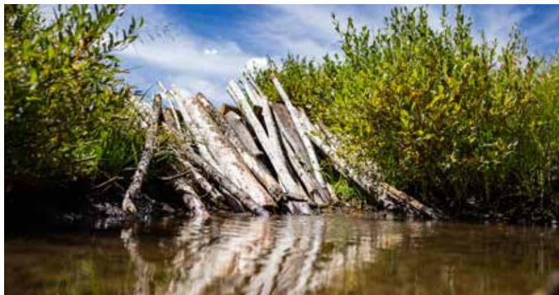
The Soda Creek in Lieu Fee Restoration site just days after the initial installations of beaver dam analogues and other instream structures. The structures act as “speed bumps”, causing the water to slow and wet the surrounding riparian habitat.
