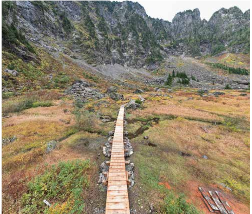
A new puncheon boardwalk on the Lake 22 Trail on the Mt. Baker-Snoqualmie National Forest.
