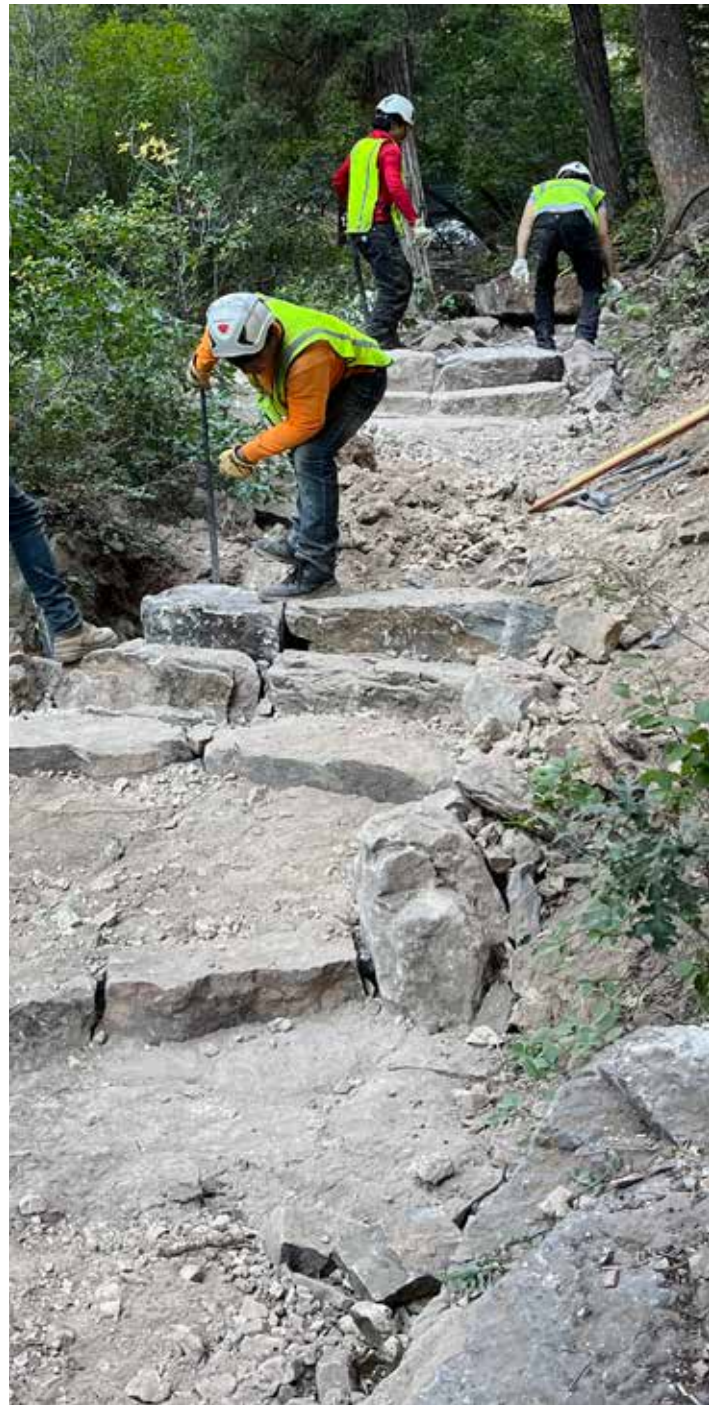
Stone masons put the finishing touches on the reconstructed Hanging Lake Trail in Glenwood Canyon, Colorado
