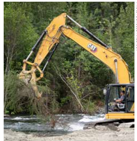
An excavator creates a new channel in Resurrection Creek.
