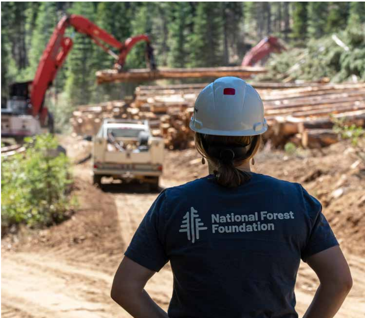
NFF's Central Sierra Program Coordinator, Anne Graham, watches as timber from the Cabin Creek Forest Health Project is sorted and prepared for transport to a lumber mill.
