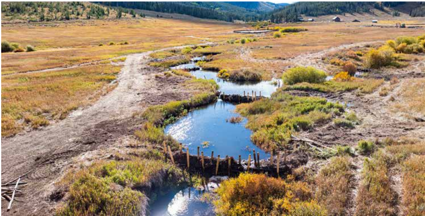
The Soda Creek in Lieu Fee Restoration site just days after the initial installations of beaver dam analogues and other instream structures. The structures act as “speed bumps”, causing the water to slow and wet the surrounding riparian habitat.
