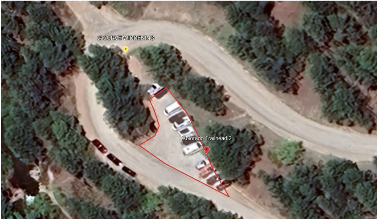
Colorado Trailhead 2 – Maintain surface, compact and surface with 3 layers of \frac{3}{4} " chip and seal. (4,000 square feet)
